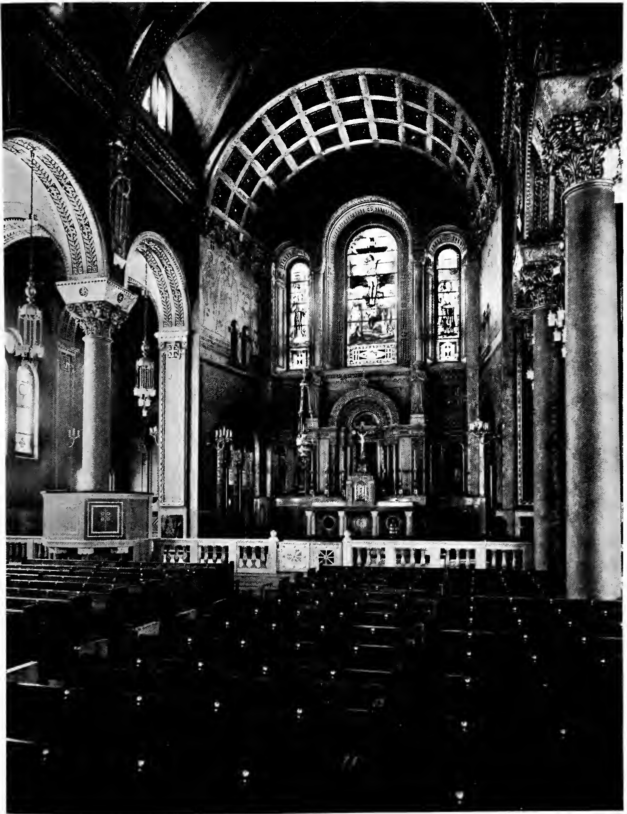
ST. JOHN'S CHURCH, NORTH CAMBRIDGE, MASS. MESSRS. MAGINNIS, WALSH & SULLIVAN, ARCHITECTS
